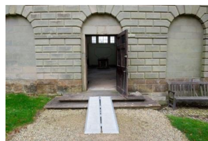
Ramp access to Chapel
